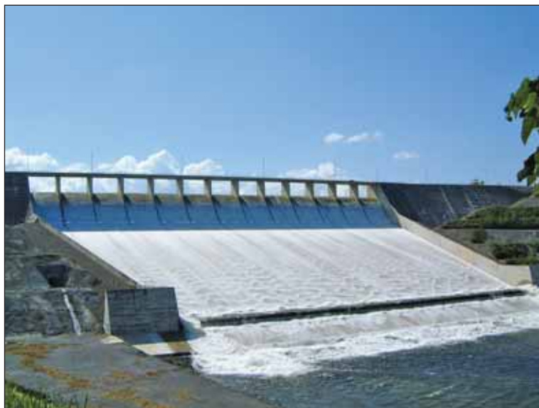
View of the Urra spillway before the Fusegate installation.
