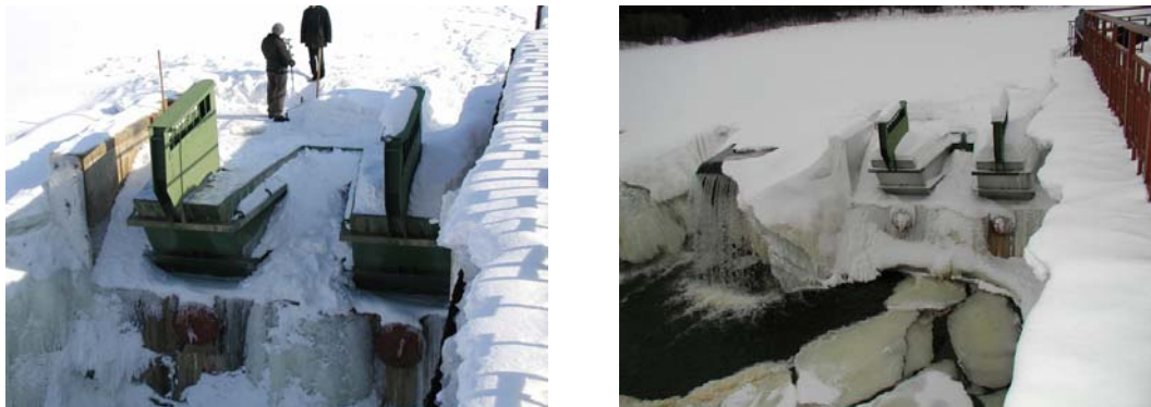
Fig. 10 Downstream view of fusegates in Winter
