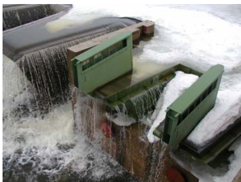
Fig. 11 Fusegate during snowmelt
