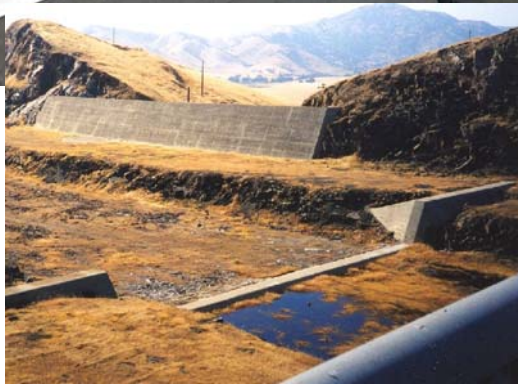
UPSTREAM VIEW OF THE SPILLWAY BEFORE REHABILITATION
