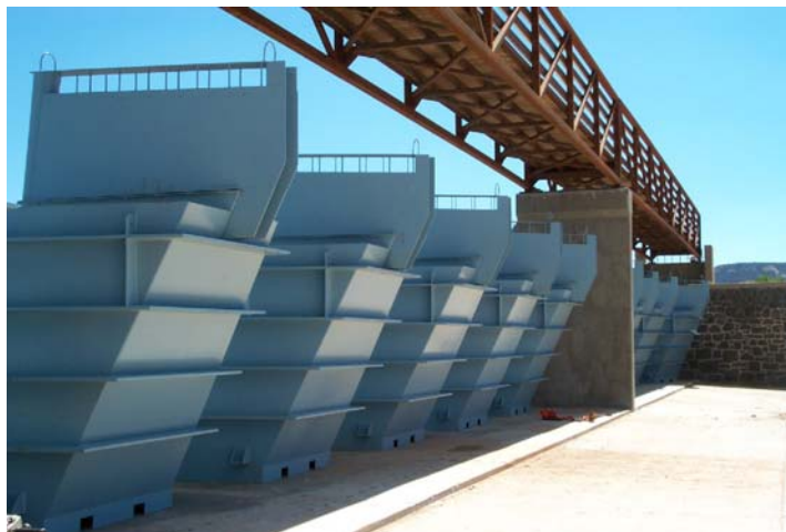
BLACK ROCK DAM, NEW MEXICO
