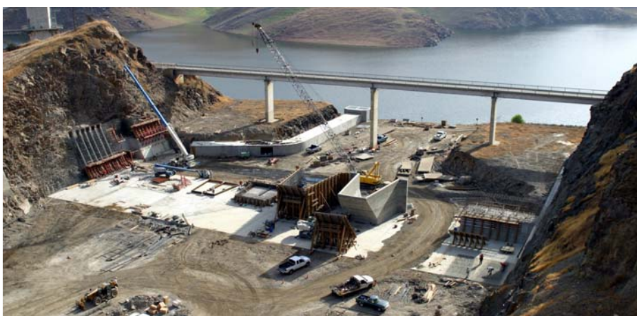
DOWNSTREAM VIEW OF THE SPILLWAY
