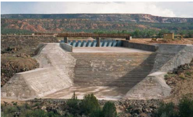
Downstream view of spillway equipped with Fusegates
